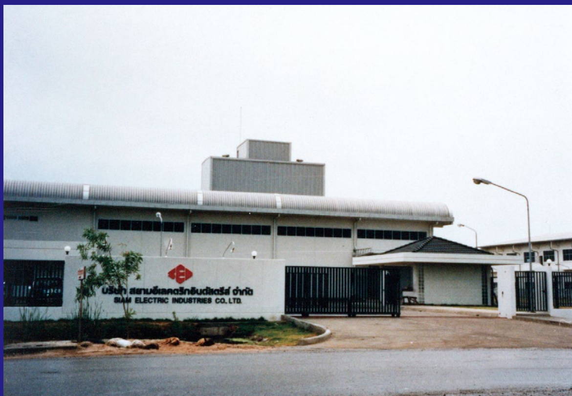
Siam Electric Industries Co., Ltd.
